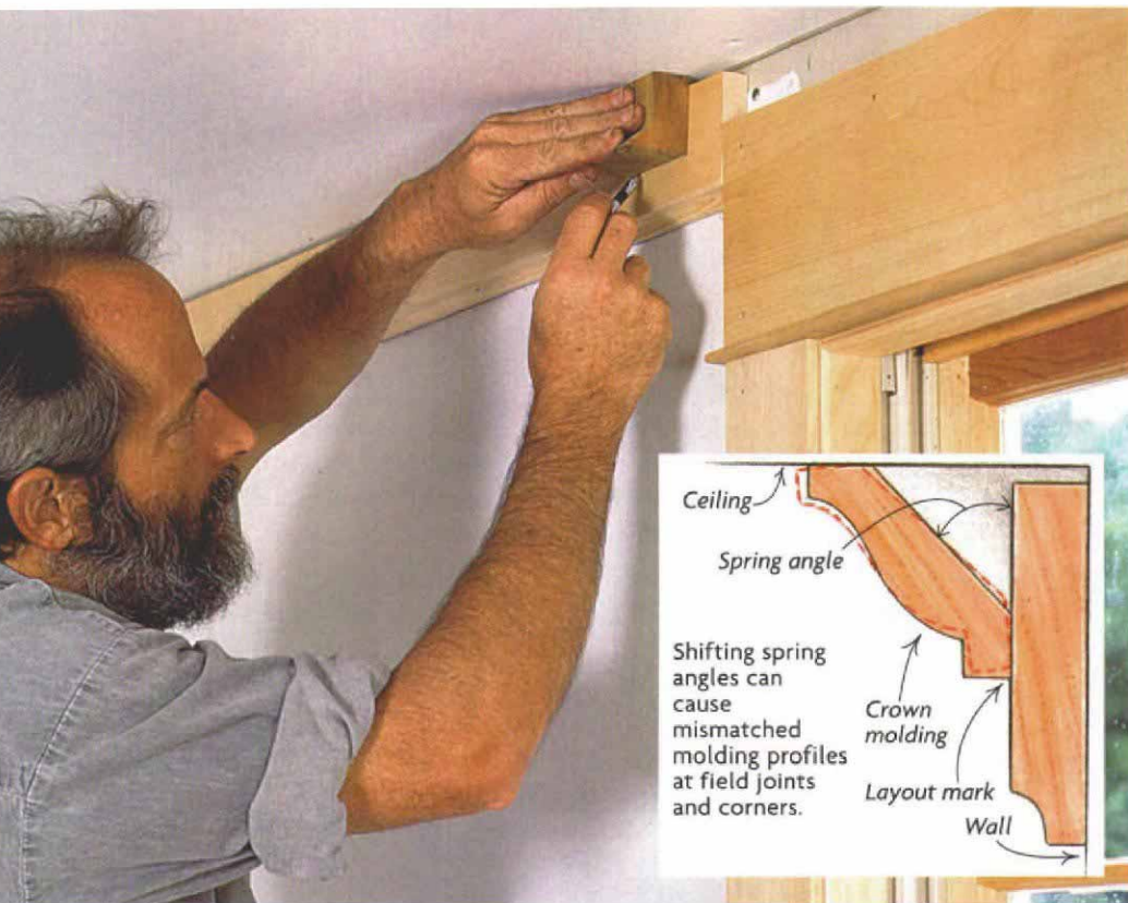
Gauge block shows exactly where the bottom of the molding must lie. Layout marks keep molding at a consistent angle to the wall, which in turn makes miters and field joints line up.
